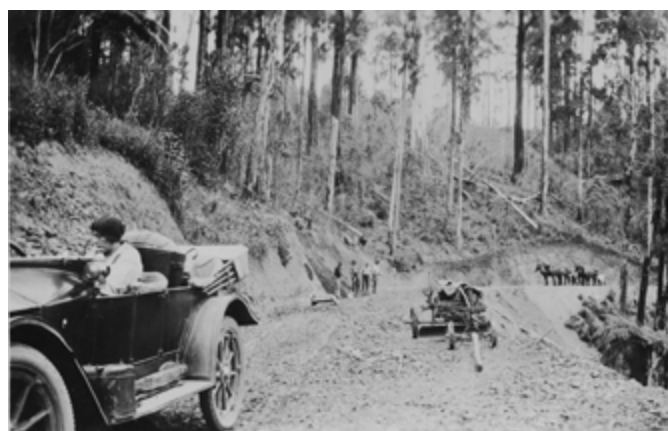
Road worker on Wild Dog Creek Road. Photo showing the Hup, my mother, and a road machine – possibly a grader, and a team of horses
