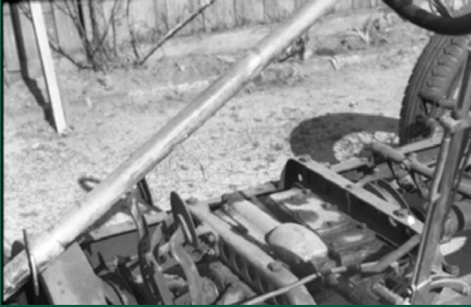
Pedal configuration and gearbox of Benz
