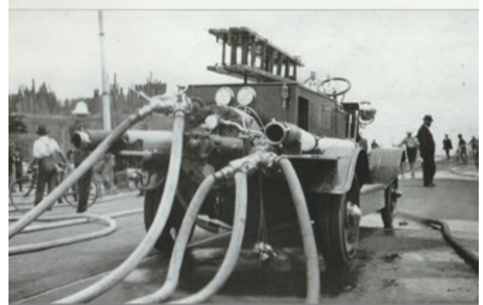
Dennis/Gwynne Turbine Pump in action a timber yard fire in Caulfield in 1919
