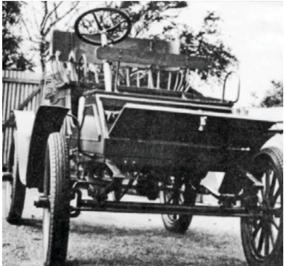
The steam car of the 1900/01 period, which was used at the Finlayson works, is seen here after its restoration in the early 60s when it was fitted with "modern" tyres. The fold out footboard, used for front seat passengers when required, is clearly visible.
