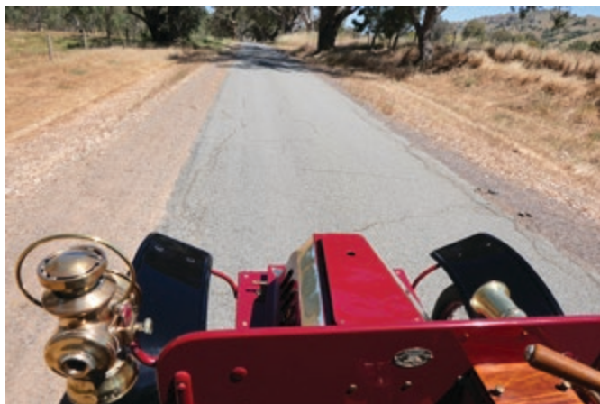
Proof of a 'well flattened' road, following the 'dashing away with a smoothing iron' efforts by our Rally Directors.
