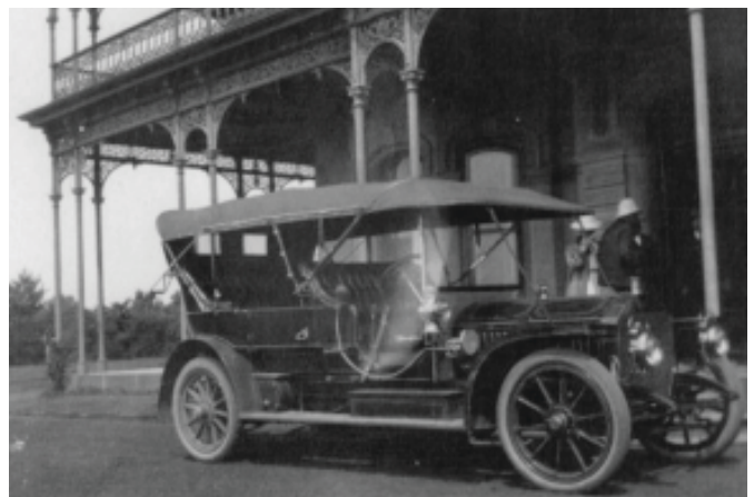
The Manifold's chain-driven, fully imported c1904 60 HP 6cyl. Napier beside "Talindert" Homestead, Camperdown.
