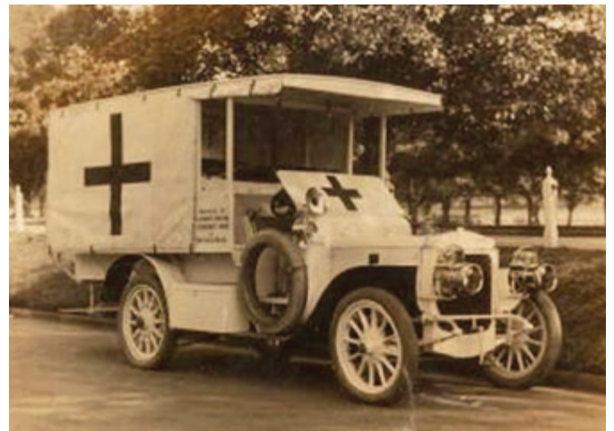
An Australian body was built for this Daimler ambulance presented by the Woman's Christian Temperance Union of New South Wales. The motor body builder is not identified but probably a firm in Sydney where the photograph was taken. The construction is the same as an ambulance body built by the Adelaide firm of Duncan & Fraser. It is likely both were constructed to the requirements specified by the military authorities. This image is from the State Library of South Australia [B56727] but appears to be reproduced from a photograph by Crown Studios, Sydney, held in the Sydney Powerhouse Collection of the Museum of Applied Arts & Sciences.
