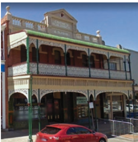
Crone's Buildings, 80-84 Napier Street, St Arnaud
