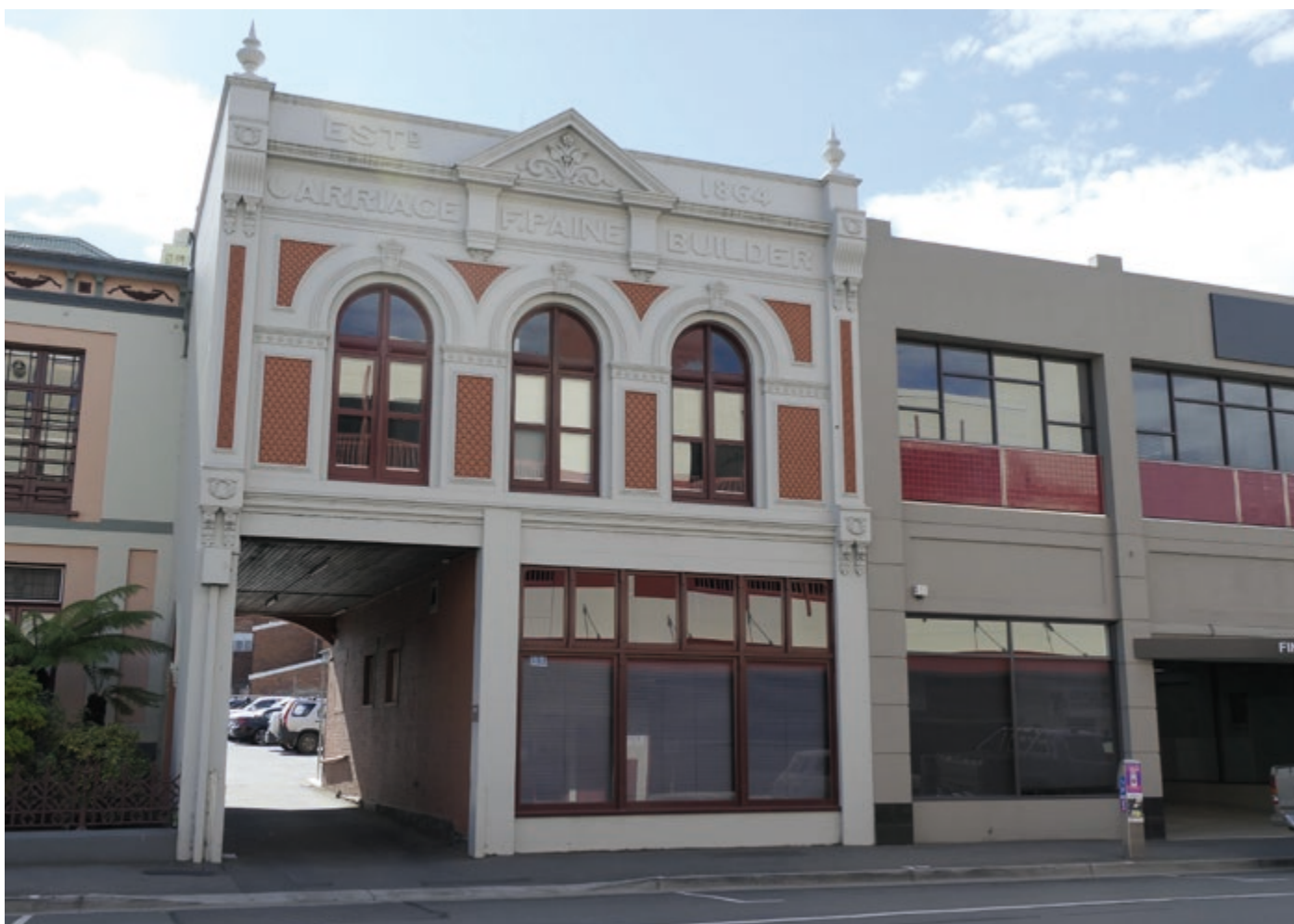
Paine Carriage Builder building as it stands today.
