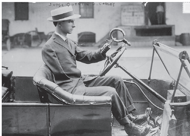
Judge Corley – adaptive steering wheel for Model T Ford
