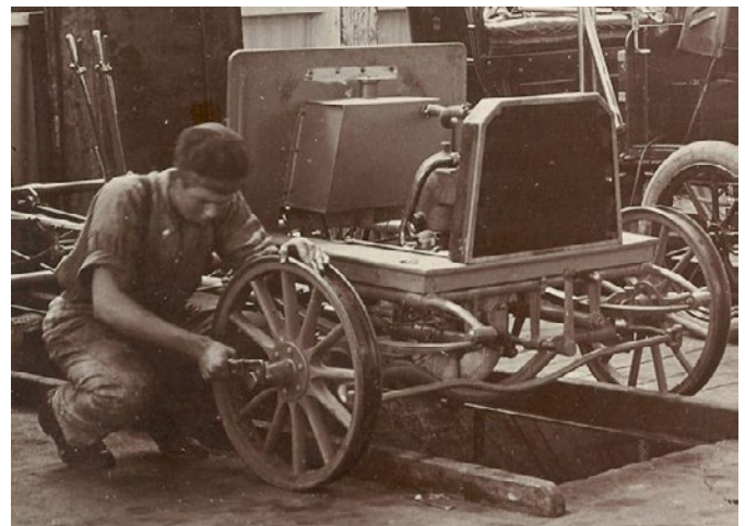
This Type 3 Lacoste was sold in Adelaide as a Lewis. Note the dropped sub-frame suspension brackets
