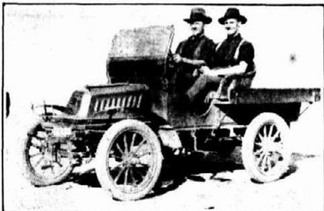
This 21-year-old De Dion Bouton, owned by Mr C. E. Woods, of M'Ilwrick street, Windsor (seen at the wheel), has run three-quarter of a million miles and carries about 7 cwt. It does 40 miles to the gallon.—“Herald.”
