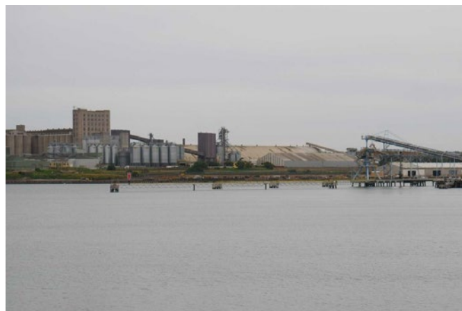
Corio Quay at Geelong Port, where the new Spirit of Tasmania Victorian berth is to be located
