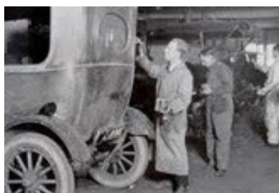
This 1923 photo shows Charles Jeffrey, an instructor at Master Motor Coach Refinishing of Detroit, using the latest technology in automotive refinishing: paint brushes. Back then, cars were sanded with gasoline between brush-painted coats and then polished with emery cloth. Photo courtesy of PPG.
