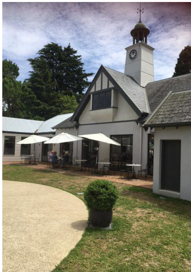
The motor house at Coombe Cottage
