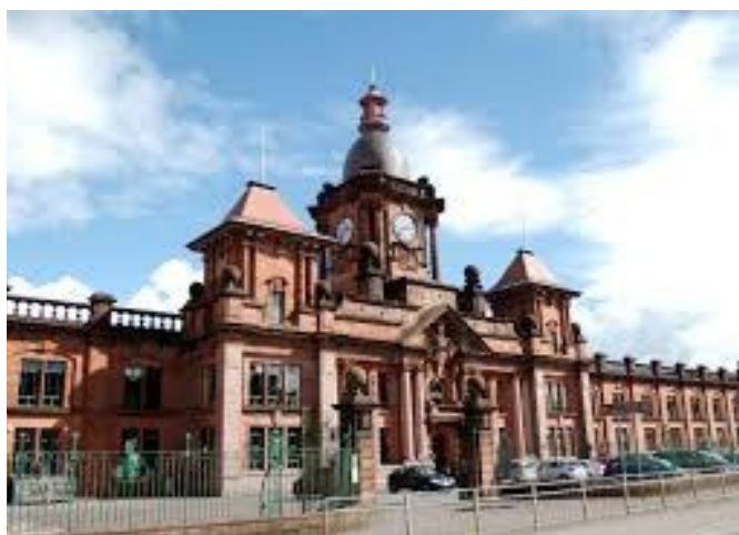
The Grand Argyll Factory facade
