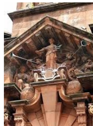
Detail of Argyll Factory Facade.
