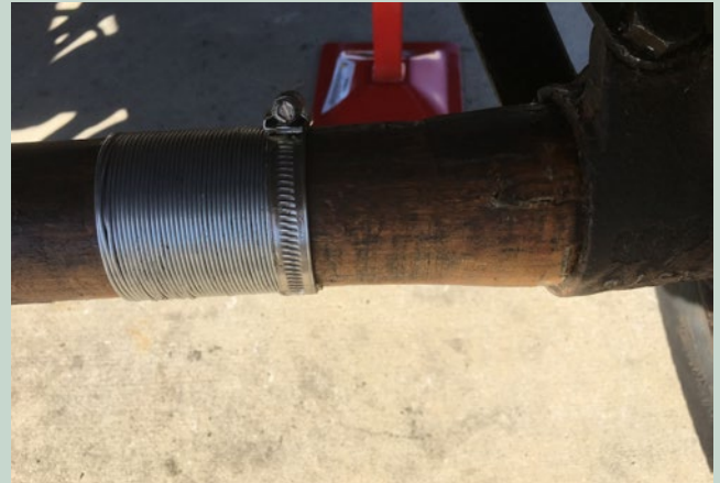
The initial axle 'bandage' did not work adequately.
