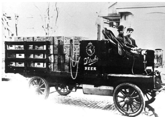
An electric wagon used for beer delivery in Detroit (1906)
